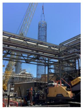
mass excavation once they were in place. "The original and more efficient plan was to mass excavate prior to pile installation as the varying elevations of each pile cap, but because of the earlier shaft redesign we had to flip the plan and install everything from grade and then go back and excavate afterwards. Because of the way the site was set up, we couldn't get equipment down there. We had to pivot."
